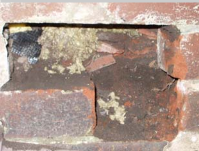
Where a visual inspection does not identify the cause, small parts of the building may have to be 'opened up'.
