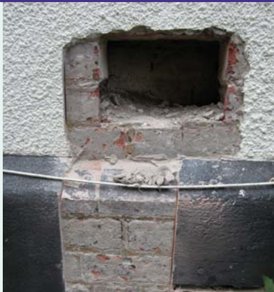
Where a visual inspection does not identify the cause, small parts of the building may have to be 'opened up'.
