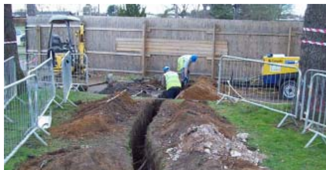
Root barrier installation in a root protection area (Landscape planning Ltd)
